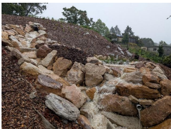
Stormwater structure at the end of Clarence Rd
